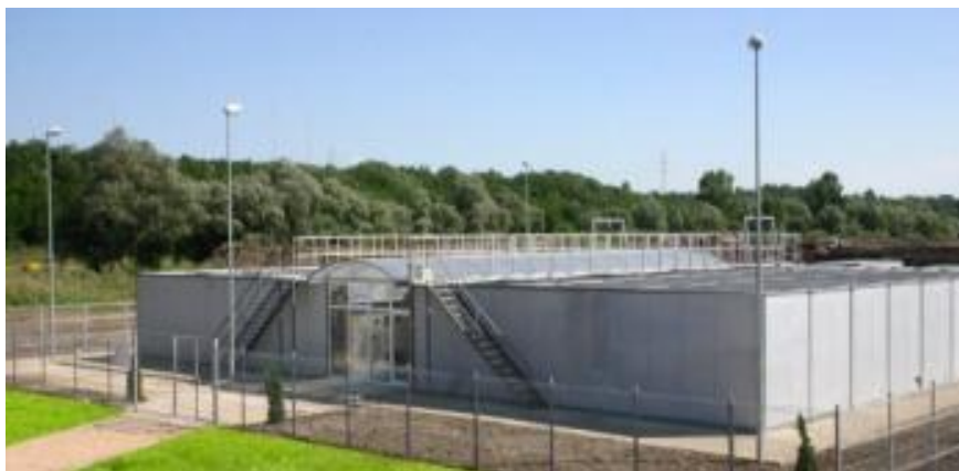
Picture 4. STP built with modules
